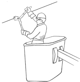
Fig. 2. A line worker crimping a compression connector with a manual compression press from a bucket (EPRI, 2001).
